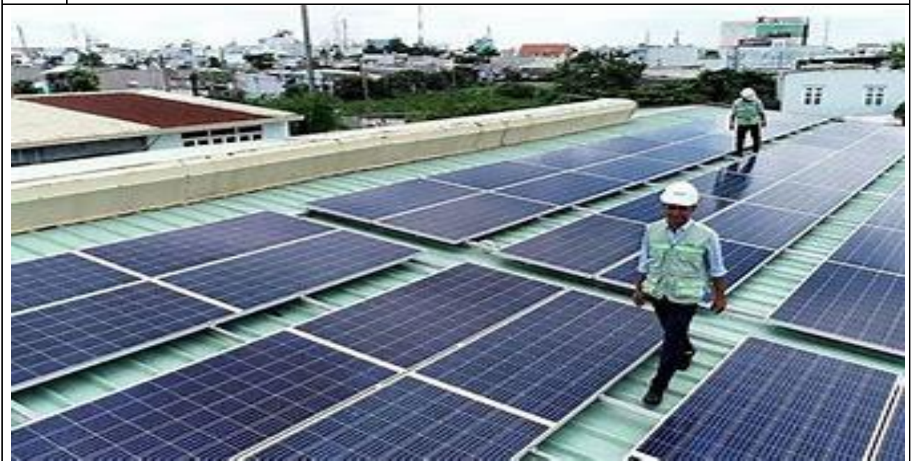
Figure 2 : Rooftop Solar Photovoltaic system
