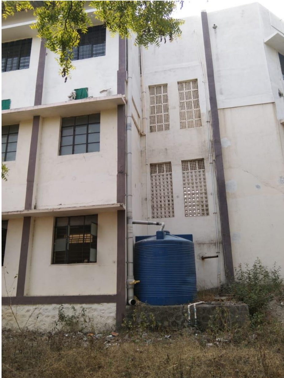
Rain water harvested at Tank
